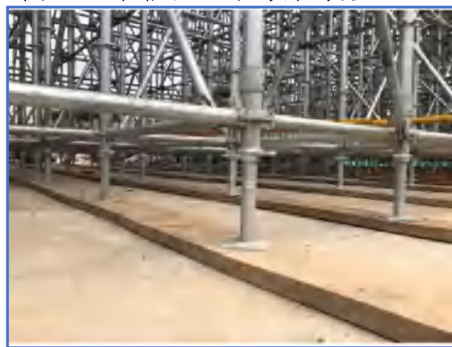
图3-10 承插型盘扣底托设置 (2)
