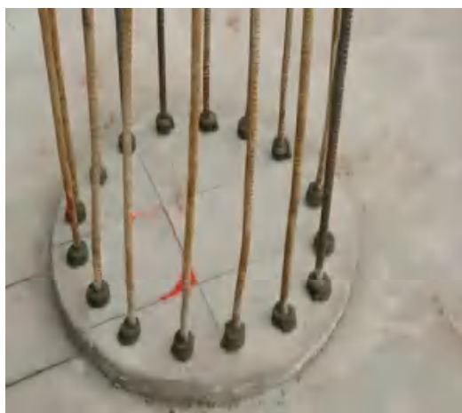
桩顶安装遇水膨胀止水条
